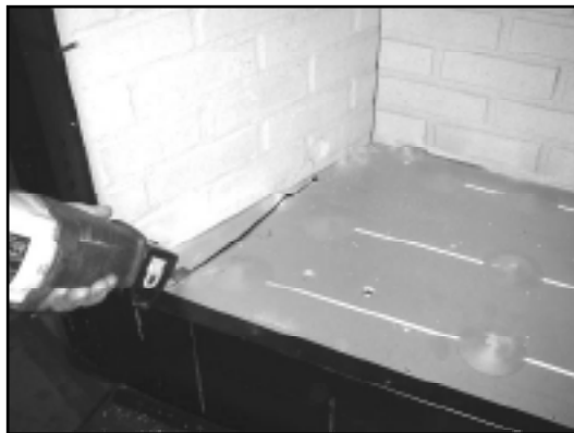
Figure 11.2. Using a saws-all, cut out the floor.
